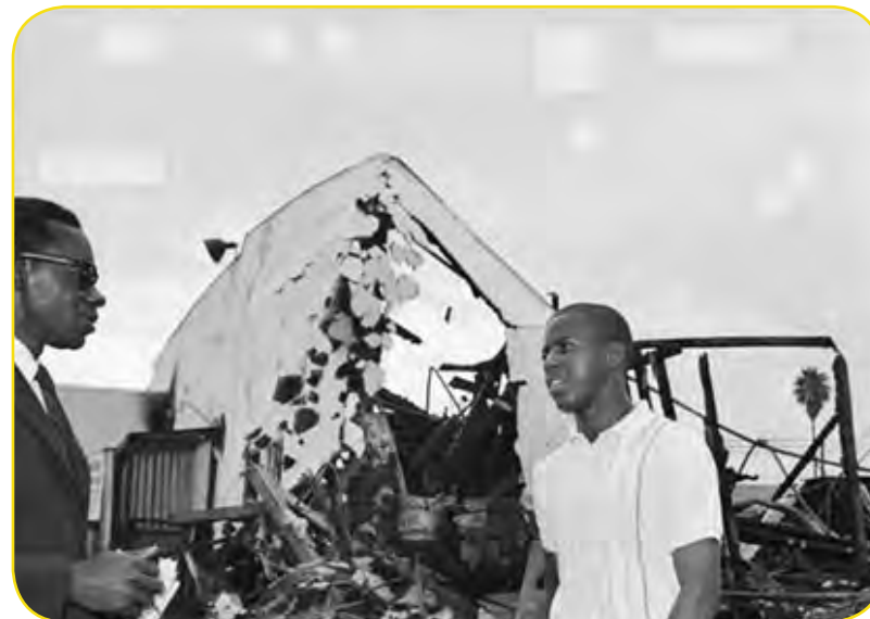
Burned residence from Watts Riots, Los Angeles, 1965 Photo: County of Los Angeles Public Library
