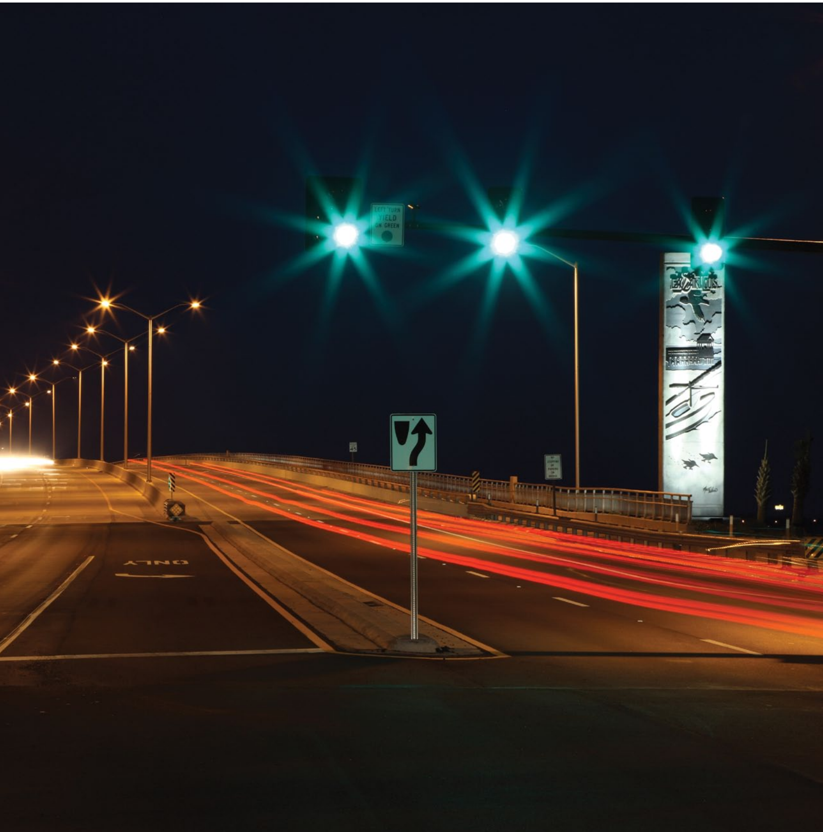
The Bay St Louis Bridge, rebuilt after the hurricane with local art incorporated into the structure. PHOTO BY JOHN THOMAS PHOTOGRAPHY
